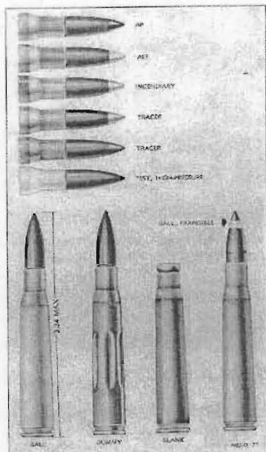
Figure 7. Caliber .30 cartridges
